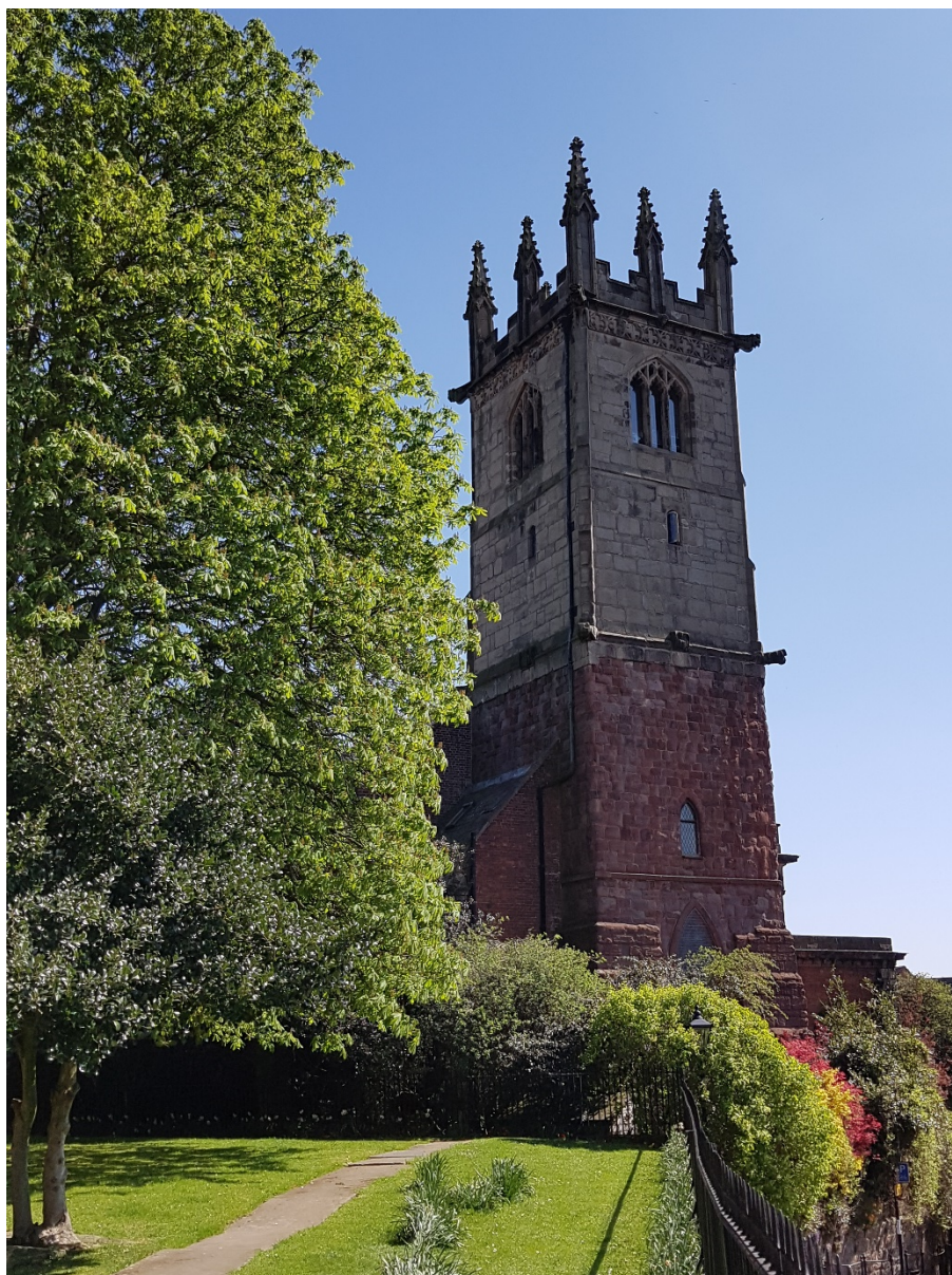
Figure 7. View of the west tower. Wendy Horton/VCH Shropshire, 2022
