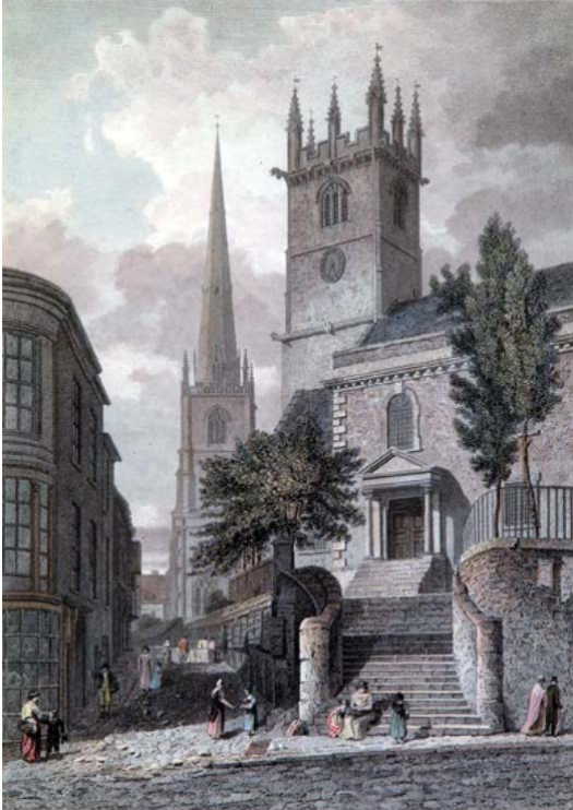
Figure 18. Entrance steps and railing, 1822. SA, SHYMS, FA/1990/26/02
